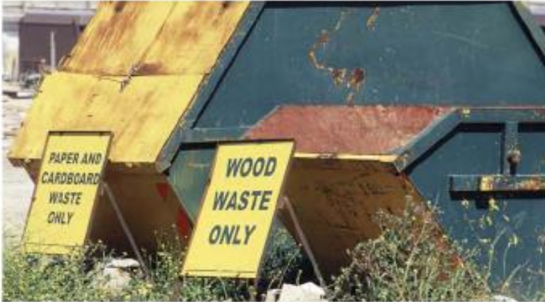
Segregated waste skips on a site for paper and cardboard and wood
