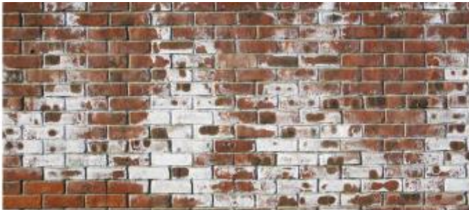
Efflorescence
